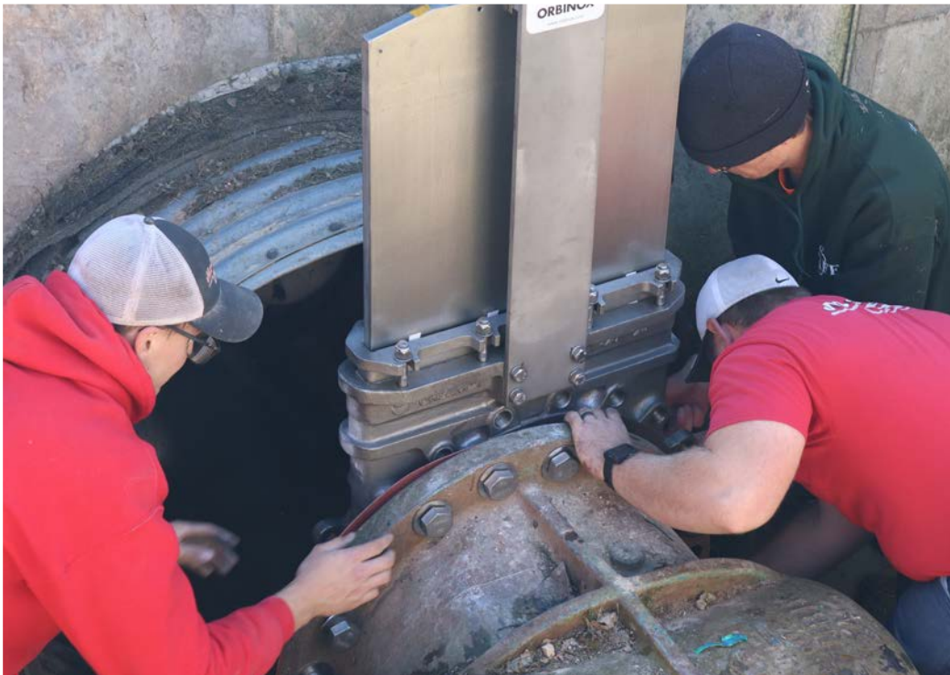
On Thursday, November 9, technicians from Molitor Plumbing, Stockton, IL and the ACL Natural Resource Manager, Tyler Hesselbacher along with assistance from the ACL Maintenance Department, installed an emergency knife valve onto the spillway valve.
