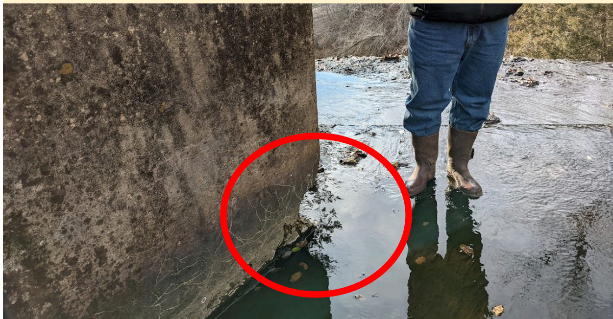
Photo: View of Plunge Pool below existing spillway discharge point
