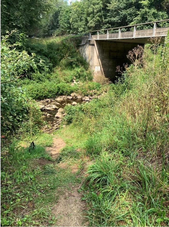
Channel downstream of bridge on South Apple Canyon Road
