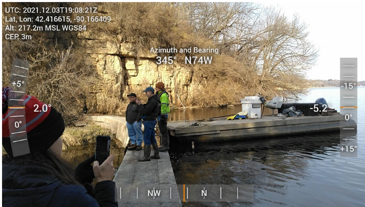
Photo: View of N-NW connection of weir wall with NW rock cut
