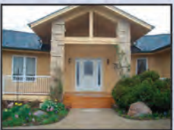
14A58 Pilot Point Lane 3 Bedroom 2 Bath Transferable Dock $319,900
