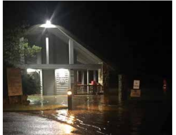
The Nixon Beach house under water.
