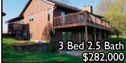
14A99 Marina View TRANSFERABLE DOCK
