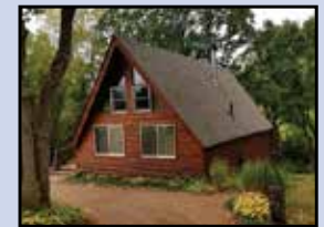
11A11 Bunker Lane 3 bedroom 1.5 Bath Transferable dock $174,900
